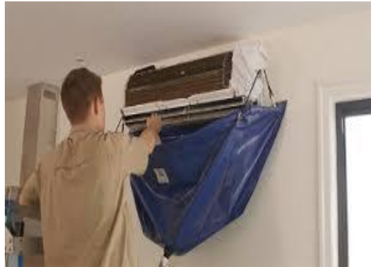
Figure 11: AC indoor unit servicing
