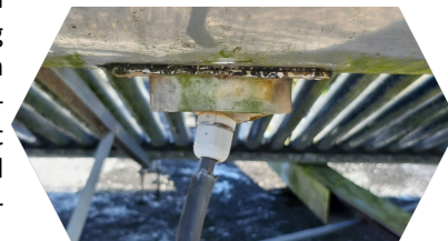
Standard Electrical booster powered with 60 V DC from direct DC solar Array.
